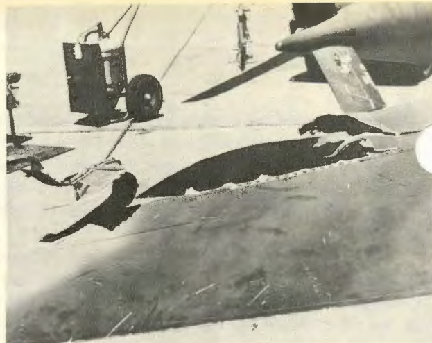
This battle damage resulted when the bombs went up and over the slab. The cause can only be classed as poor release conditions.
